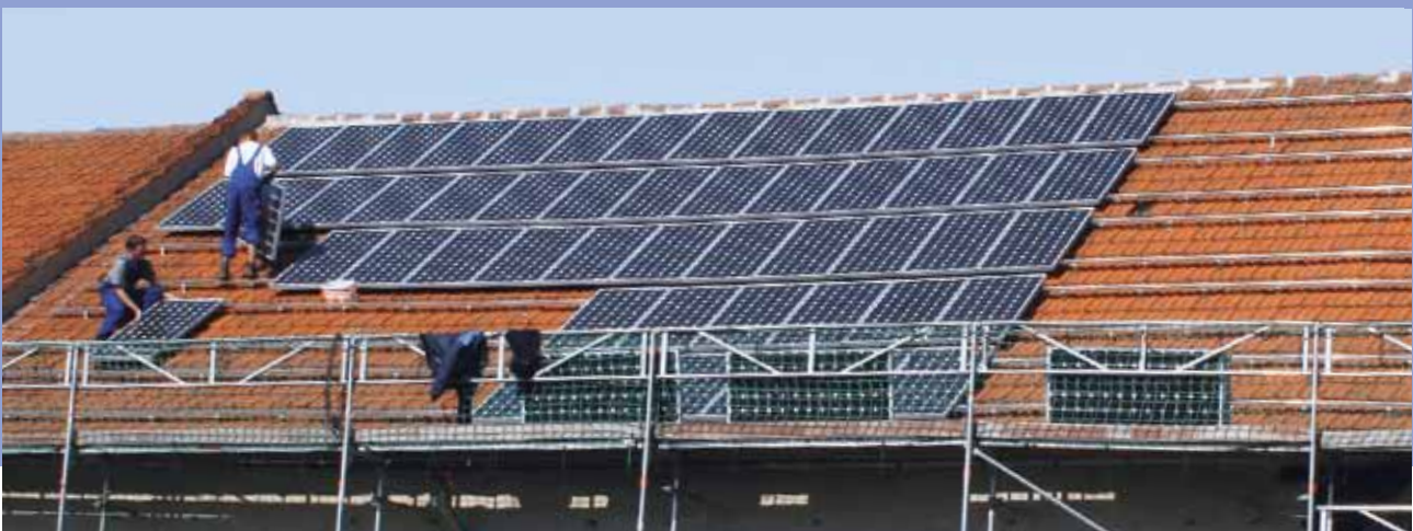
Construction with pan tiled roof hooks
