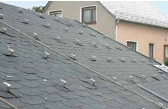
Roof with shingle roof hooks
