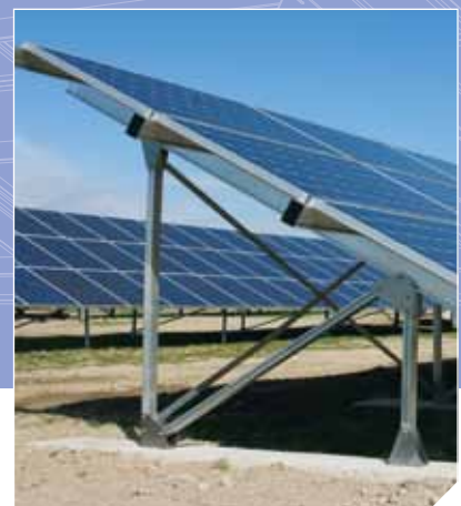
Concrete foundation
