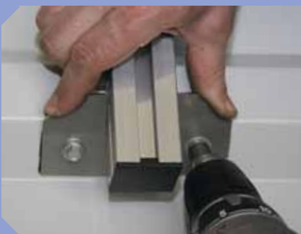
Screw connection with the roof
